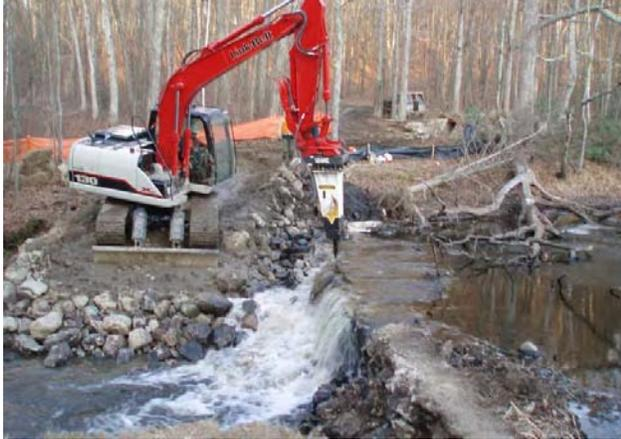
In these cases, construction is completed by drawing down the impoundment by opening the dam’s gates or creating a breach in the structure. Construction equipment enters the area along the dry stream margins or by creating an access road. Experience has shown that while there may be a temporary increase in turbidity or nutrients going down stream, these levels rarely exceed background levels or storm induced flows.
